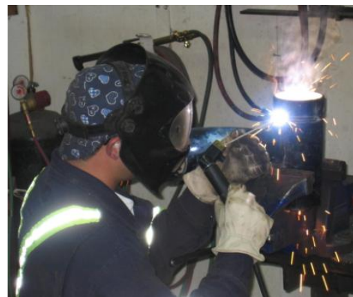
EXECUTION | Assigning pre-planned work orders, understanding progress and removing roadblocks throughout the day is key to staying on track.
